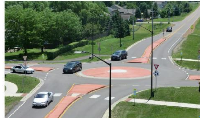
Mini-roundabout - 62' Diameter, Source: FHWA
