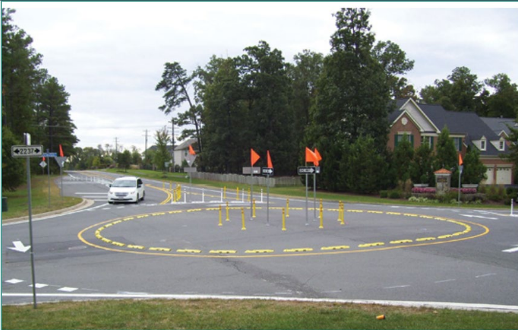
Interim Roundabout installed in 6 days
