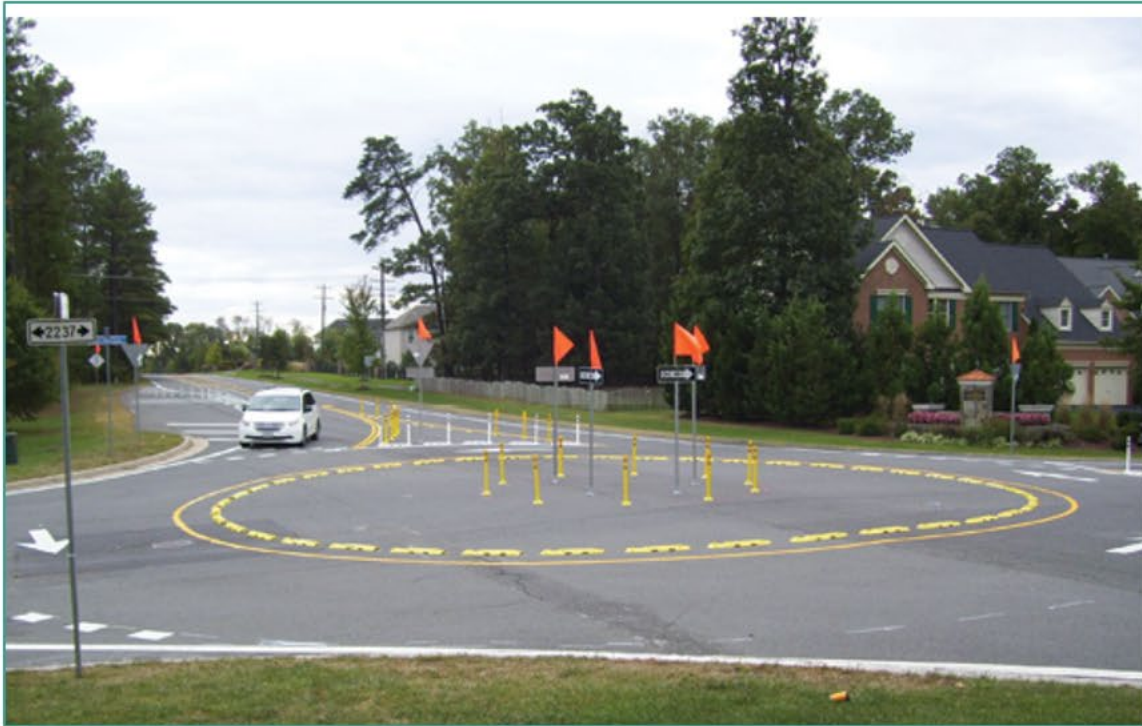
Interim Roundabout installed in 6 days
