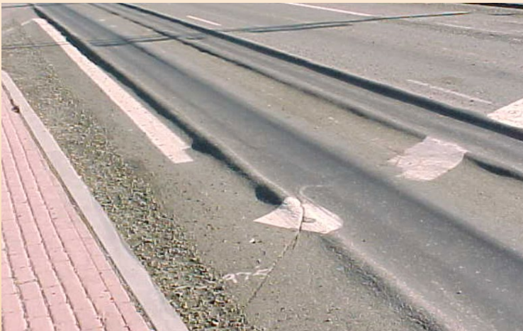
Surface Rutting of the Asphalt Concrete
