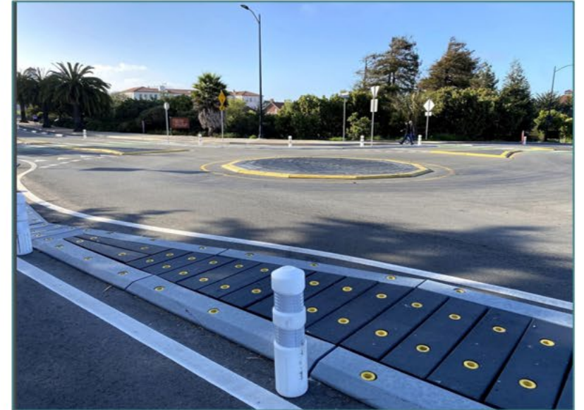
Modular roundabout pre-fabricated components curbs and islands (various sizes)
