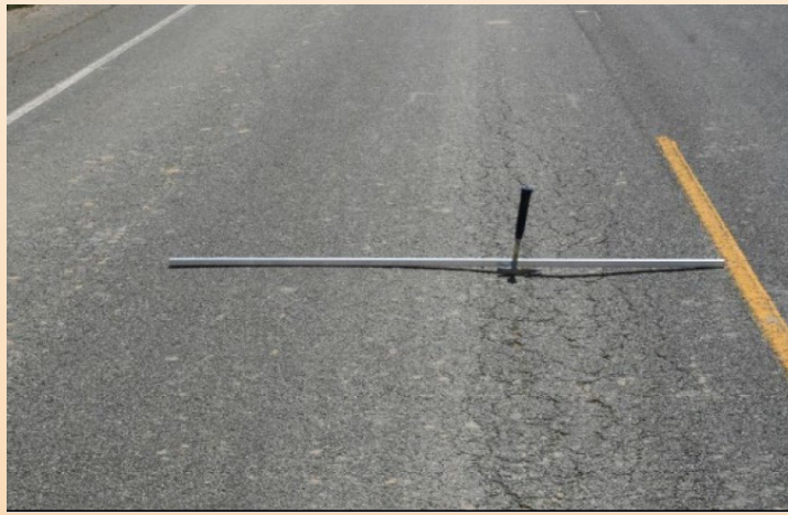
Rutting Associated with Base/Subgrade Failure
